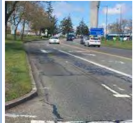
Existing Roadway Conditions
