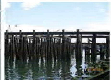
Piles prior to removal.
