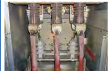
Shown here (before any cleanup) is the interior of switchgear that was protected by SEL, light-sensing and overcurrent protection during a 6.5 kV arc-flash event. Damage was limited to arcing on the cable termination bolts.
