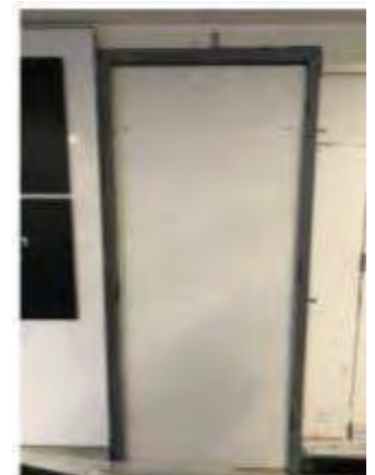
Corridor Level – New Maintenance Access Doors
